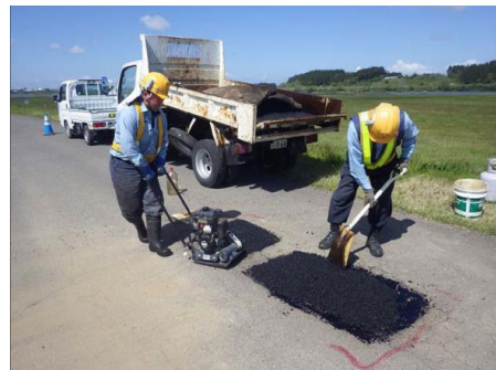
堤防天端の補修状況
